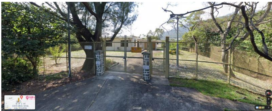
Plate 4.51: No. 52 South Lantau Road (W.S.D Quarter) in 2021 338
