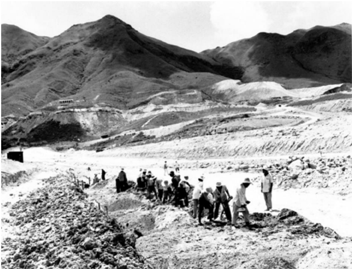
Plate 7.38: Constructing the Shek Pik Reservoir, 1961 661 .
