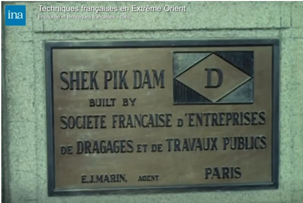
Plate 7.69: Memorial Stone of Constructor of Shek Pik Reservoir Main Dam in 1963 697
