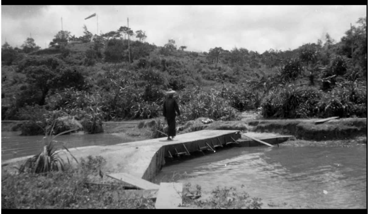
Plate 4.79: The river-crossing bridge in 1965. The pole at the top left of the phot should be the wind-sock pole mentioned in Chapter 4.8.2.1 393 .
