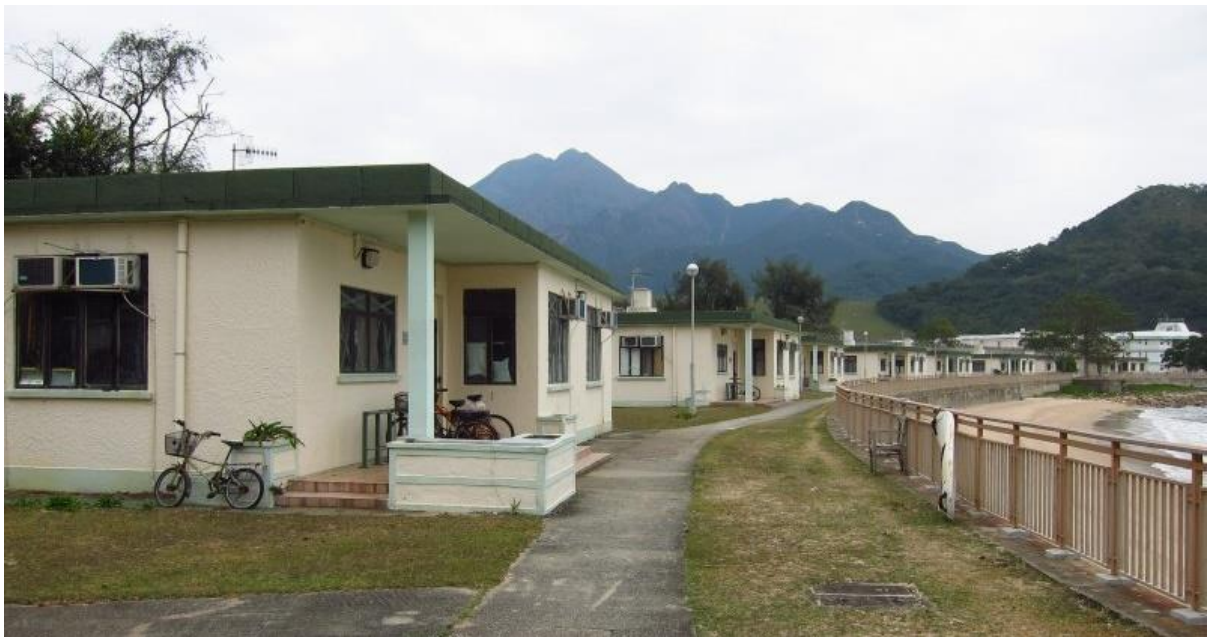
Plate 7.83: Staff quarters of Sha Tsui Correctional Institution in 2016 719
