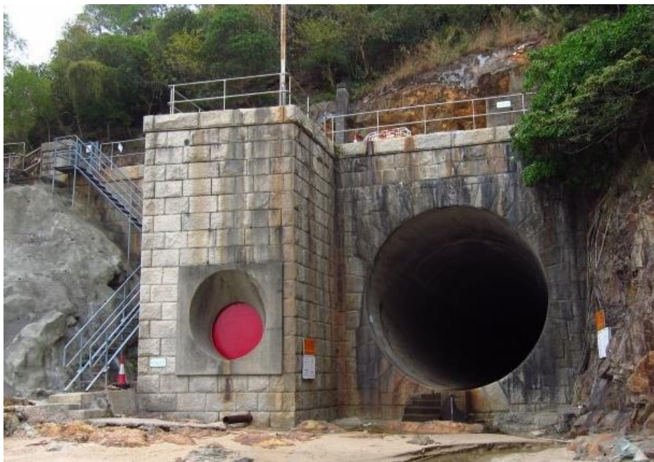
Plate 7.72: Outlet of Discharge Tunnel in 2015 699
