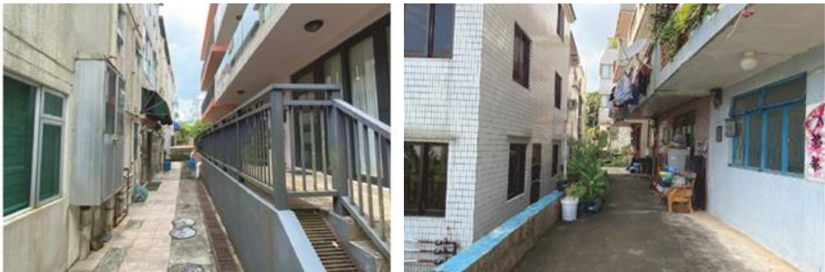
Plate 6.36: Stepped terrace (left) and shared terrace (right) of Shui Hau village houses, photo taken by the research team in 2020.
