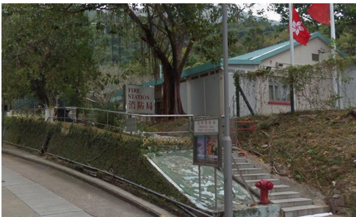
Plate 4.64: Cheung Sha Fire Station in 2016 364
