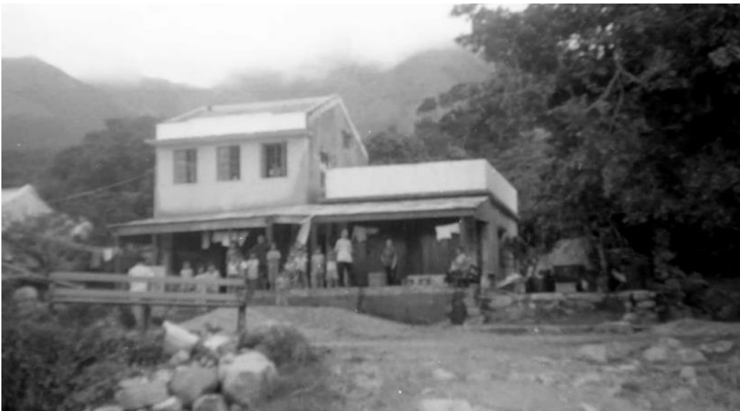
Plate 5.14: Village building at Tong Fuk Village in 1965 439
