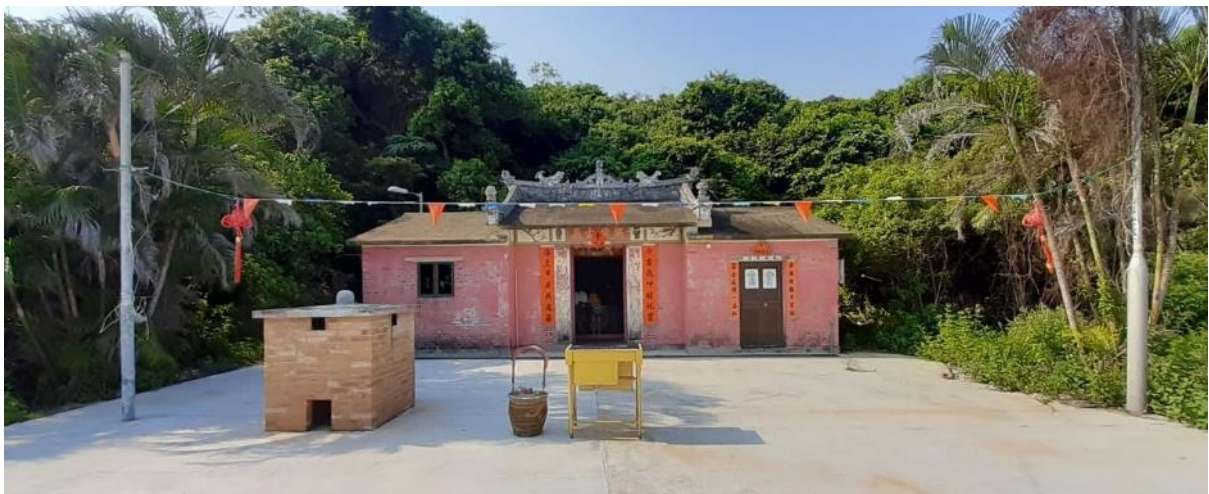
Plate 7.36: Hung Hau Temple exterior, Tai Long Wan, photo taken by the research team in 2021.
