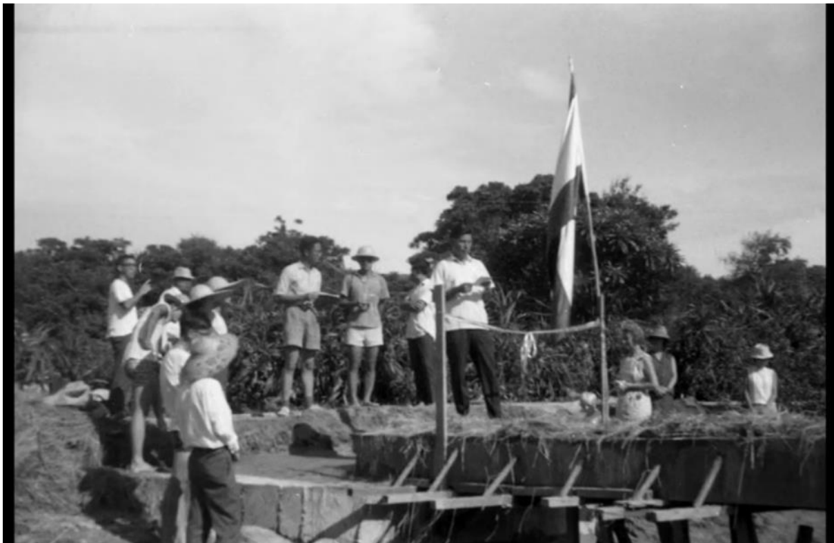
Plate 4.78: Opening ceremony of the river-crossing bridge in 1965 392
