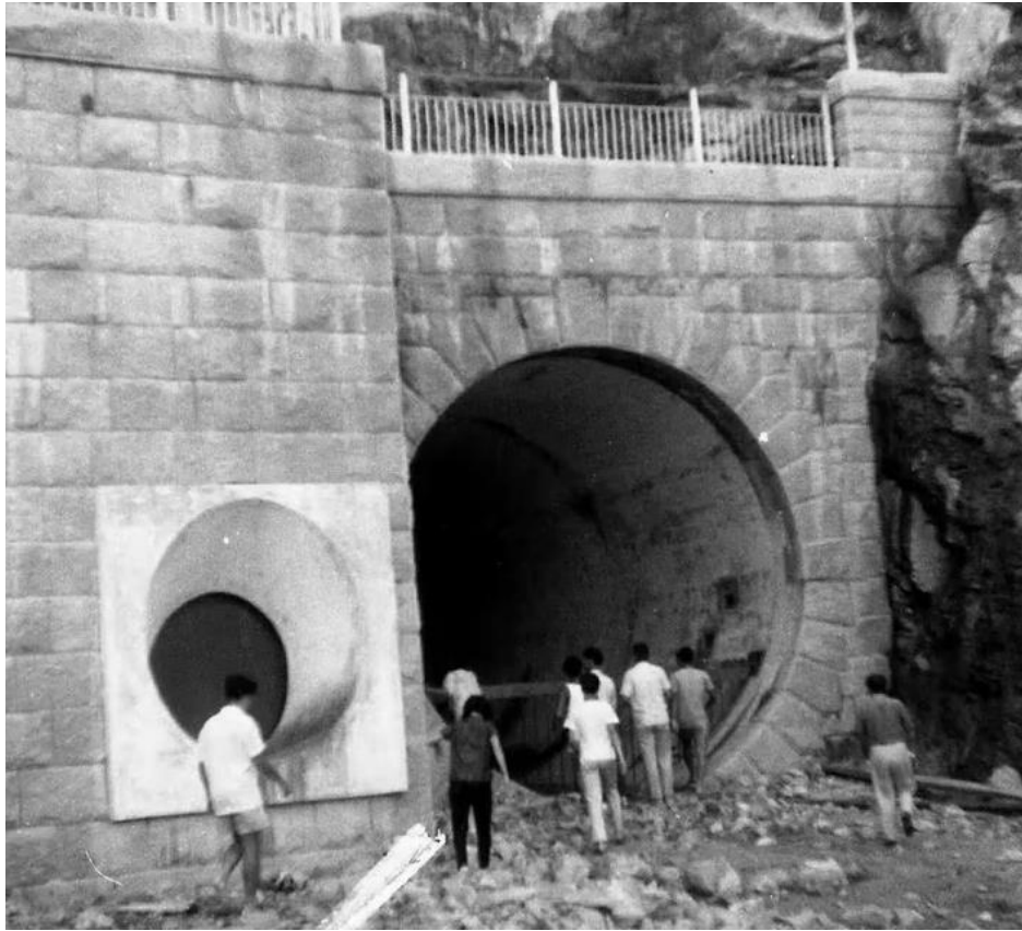
Plate 7.71: Outlet of Discharge Tunnel in 1965 698
