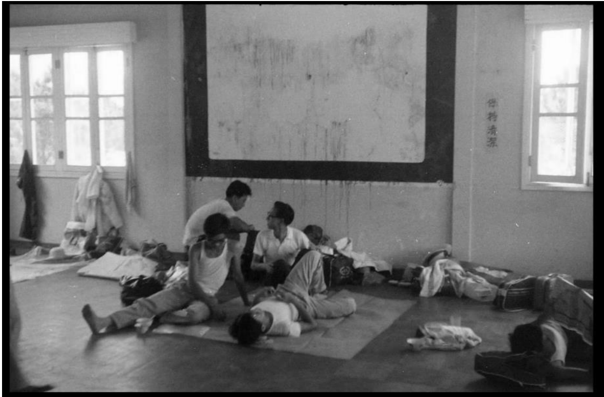
Plate 4.61: Interior of the old building of Cheung Sha Fire Station in 1965 361
