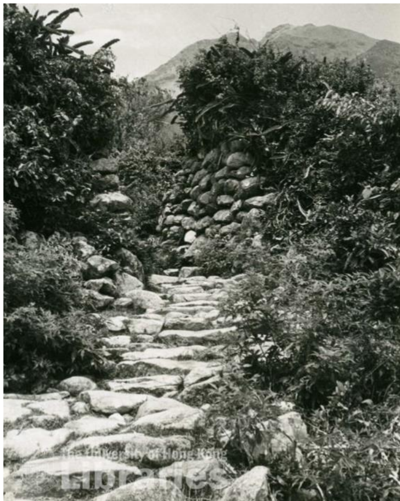
Plate 7.48: The South Gate of Shek Pik Wai. The stone wall was built by piling up big pebbles picked from the stream 676 .
